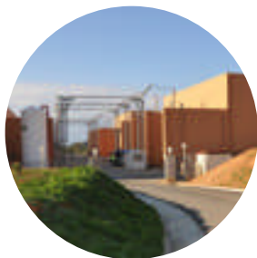
Images of equipment in the converter stations
